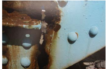
The seriously deteriorated 84-year-old Kennedy Mill Bridge on KY 152 over Herrington Lake -- closed this month for repairs -- is illustrative of the serious bridge replacement-repair problem facing the state. (Top and center photos by Gerard Gerhard. Close-up photos by Transportation Cabinet.)
