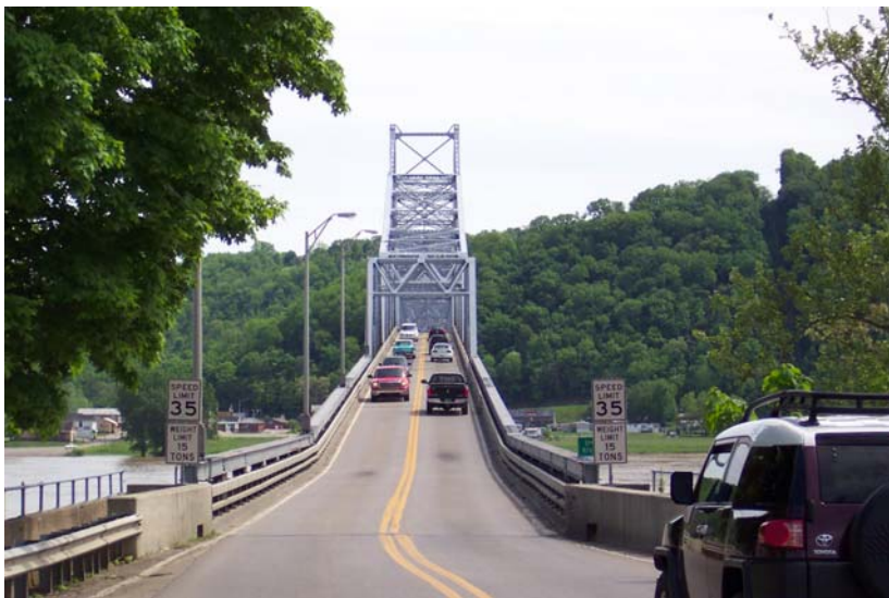
The Milton-Madison Bridge
